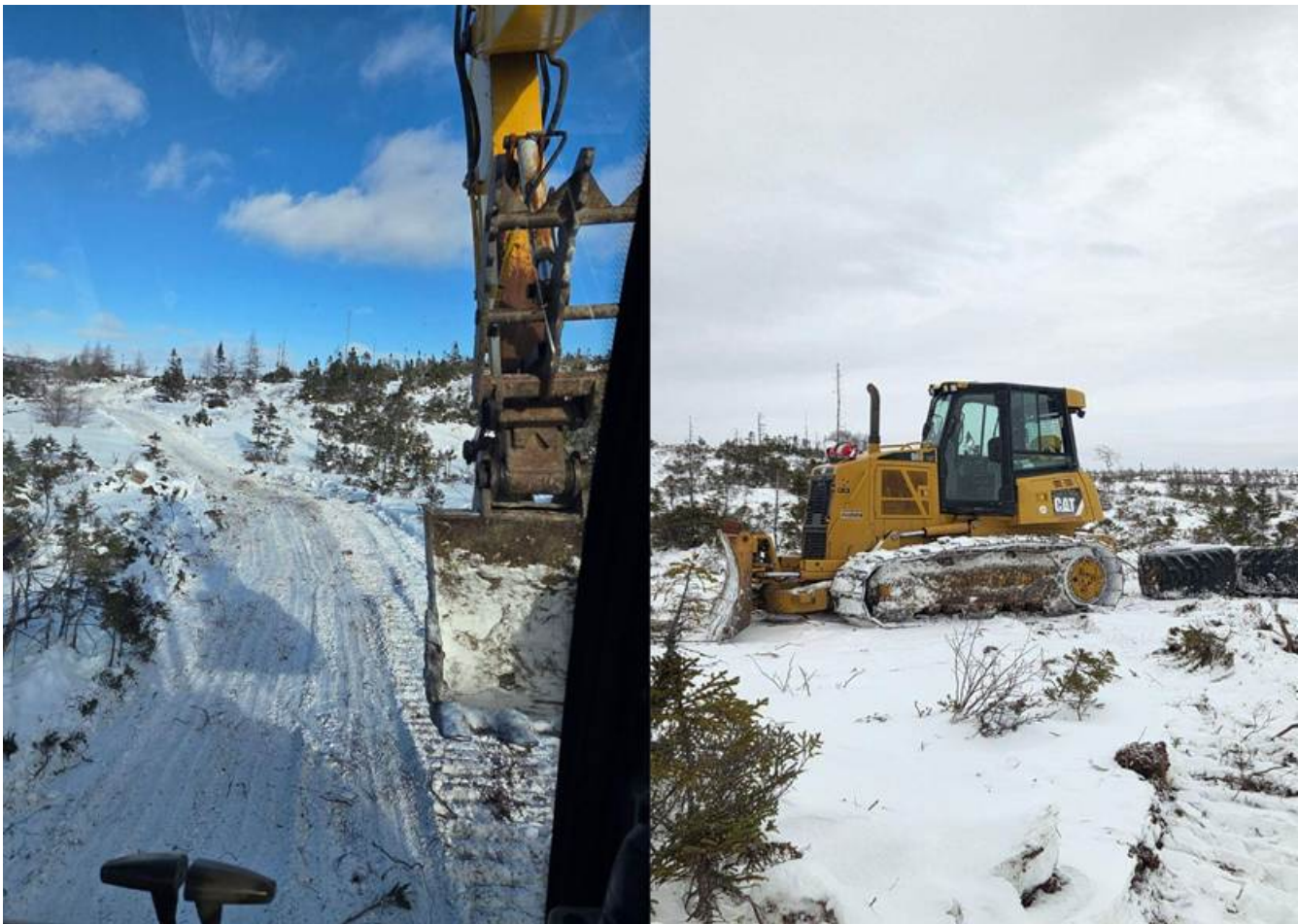
Figure 10: Drill trail construction at the Pipestone XL Awaruite Nickel-Cobalt Alloy Project, where a dozer clears brush and snow for access new drill sites for accelerated 2026 Winter drilling program; (left) tires smooth the surface for crew access by all-terrain vehicles while minimizing ground disturbance.
